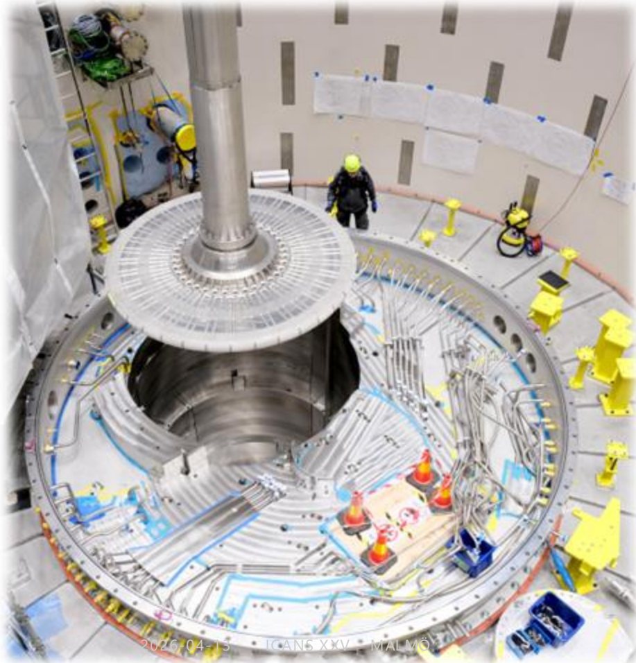
Installation of the Target Wheel
